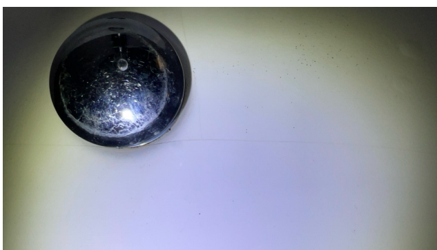
Riss i servant
