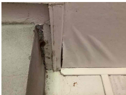
Fuktmerker i himling rundt pipe.
