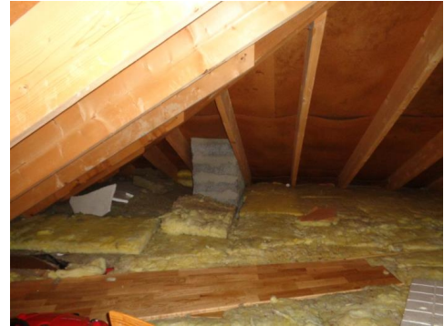
Upusset pipe i knevegg.
