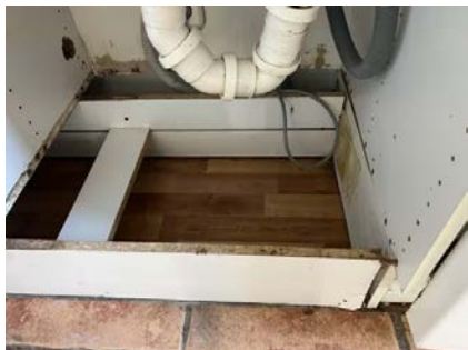
Fuktskade under vask.
