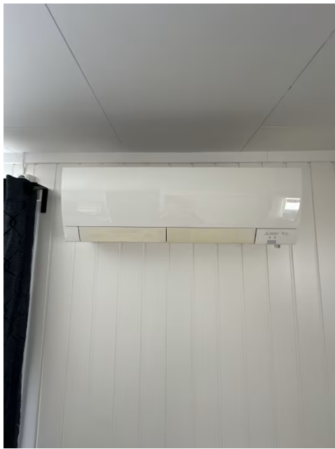
Viser innedel for varmepumpe
