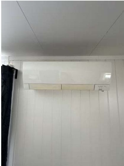
Viser innedel for varmepumpe
