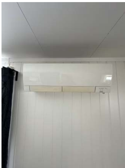
Viser innedel for varmepumpe
