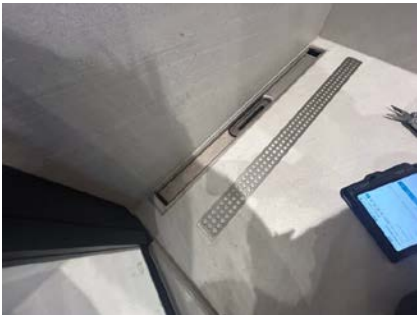
Slukrenne langs vegg
