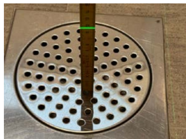
Fallforhold ca. 116 mm topp slukrist
