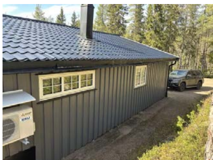
Manglende adkomst for feier.
