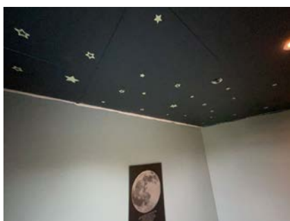
Soverom mangler himlingslister.
