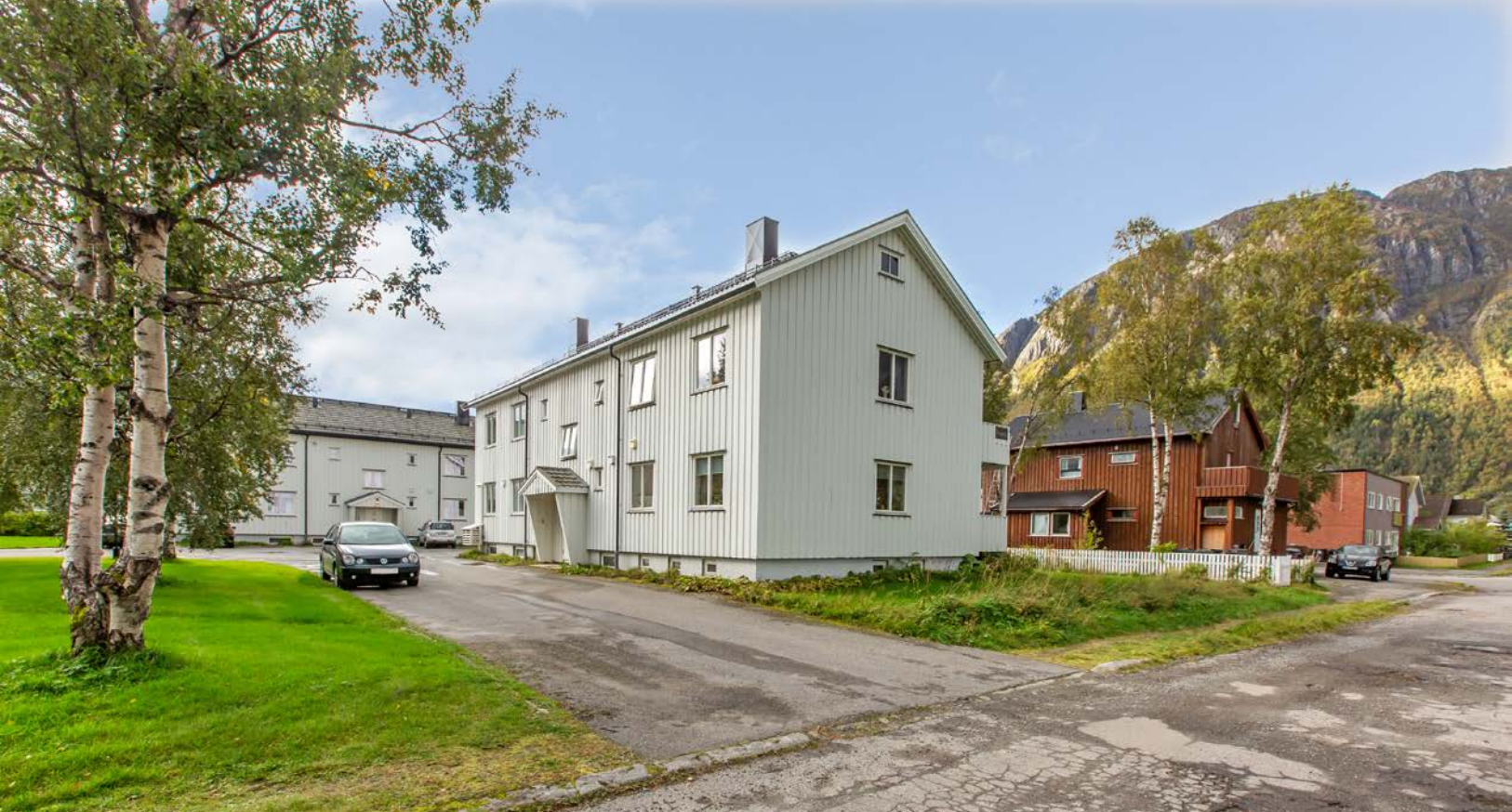
Fasade, parkering foran leiligheten
