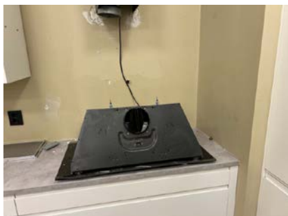
Ventilator tatt ned.
