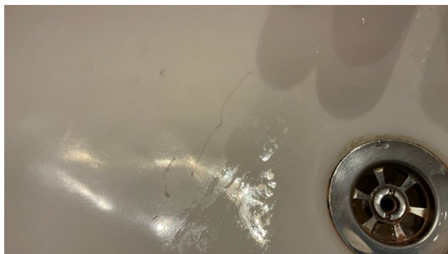
Riss i servant.
