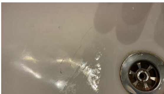
Riss i servant.
