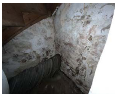
Grunnmur under trapp.
