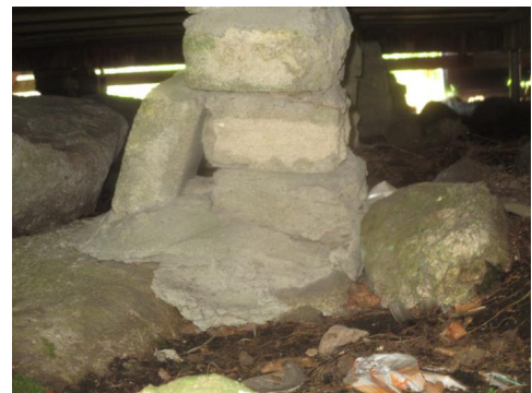
Noe enkel fundamentering.
