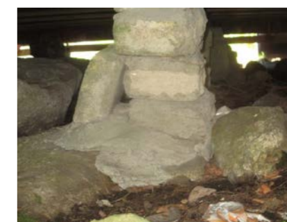
Noe enkel fundamentering.
