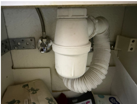
Røropplegg under servant.
