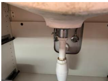
Rørprolegg under servant.
