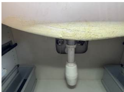
Rørprolegg under servant.
