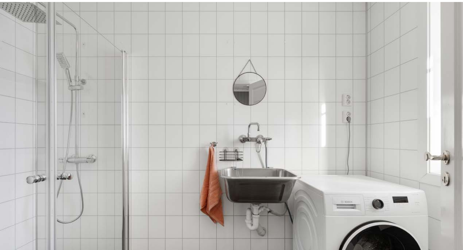
Opplegg for vaskemaskin.
