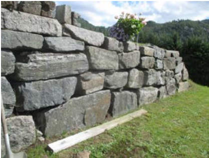
Maskinstablet mur.
