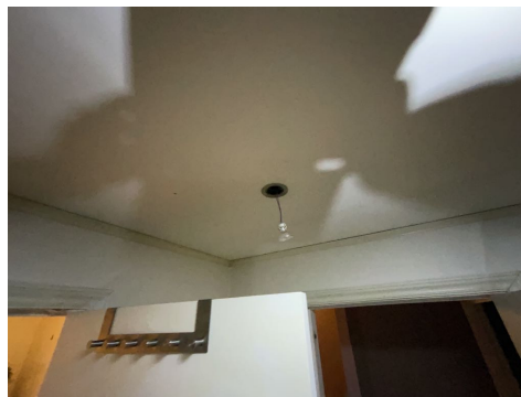
Downlight i gang.
