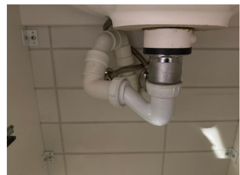
Røropplegg under servant.
