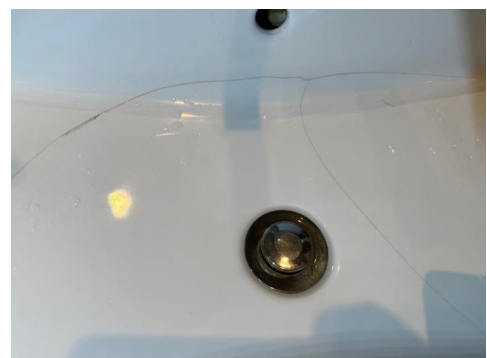
Sprekker i servanten
