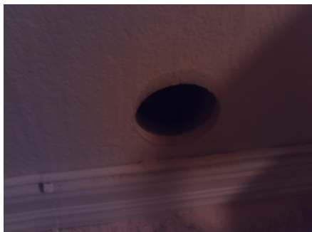
Hulltaking i utfored vegg.
