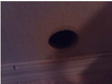
Hulltaking i utfored vegg.
