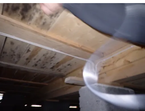
Sverting oppunder bjelkelag.
