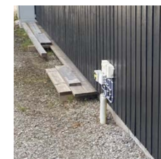
Bryterpanel for varmekabler.
