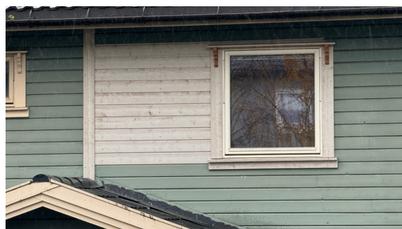
Manglende overflatebehandling.
