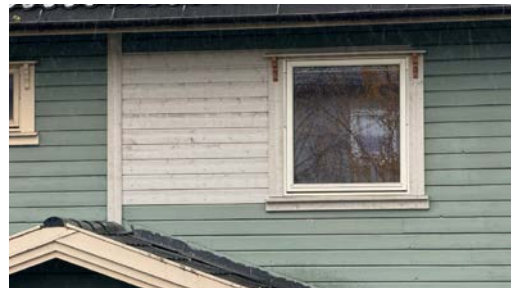
Manglende overflatebehandling.
