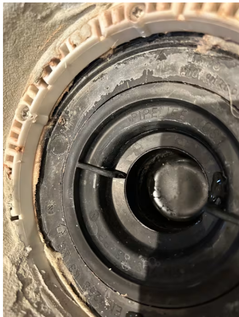
Ufulstendig membran under klemring.
