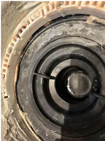
Ufulstendig membran under klemring.
