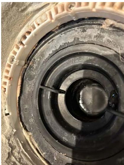
Ufulstendig membran under klemring.
