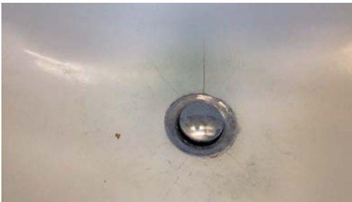
Riss i overflate i vask.
