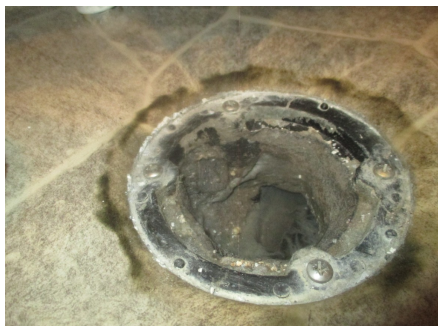
Eldre sluk under vaskekum
