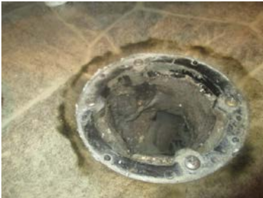
Eldre sluk under vaskekum
