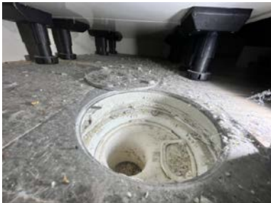
Sluk plassert under vaskemaskin
