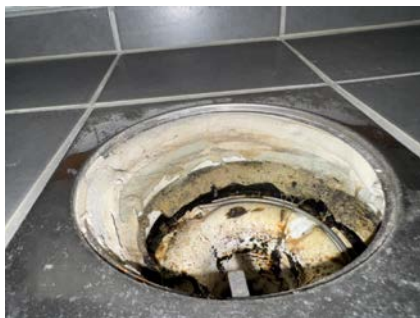
Membran klemmt ok under klemring
