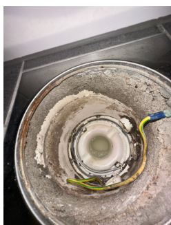
Sluk i plast, plassert under servant
