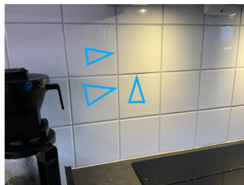
Groper i flisfuger
