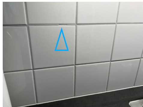
Groper i flisfuger
