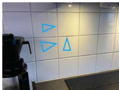
Groper i flisfuger
