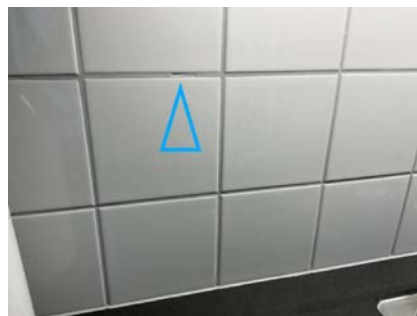
Groper i flisfuger
