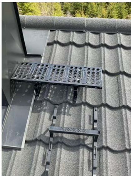
Adkomst for feiling.
