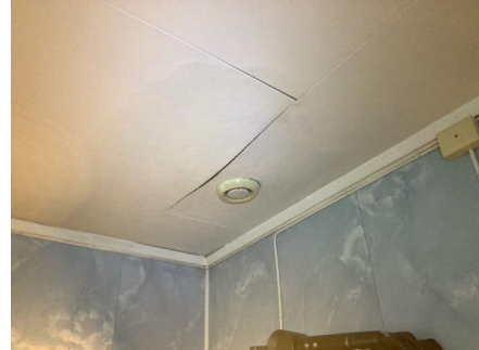
Fuktskadet himling.
