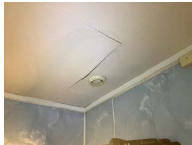
Fuktskadet himling.
