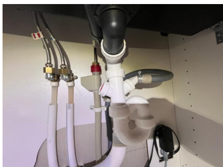
Mangler tettemuffer
