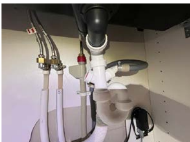
Mangler tettemuffer
