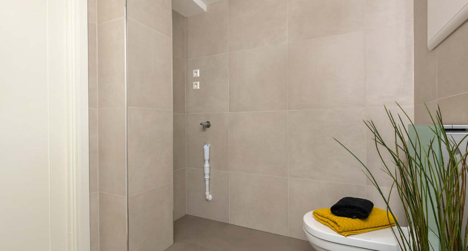
Opplegg for vaskemaskin.
