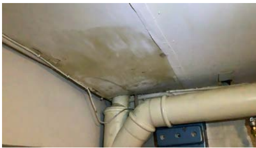
Fuktskadet himling.
