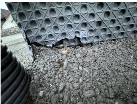
Skadet fuktsikring.
